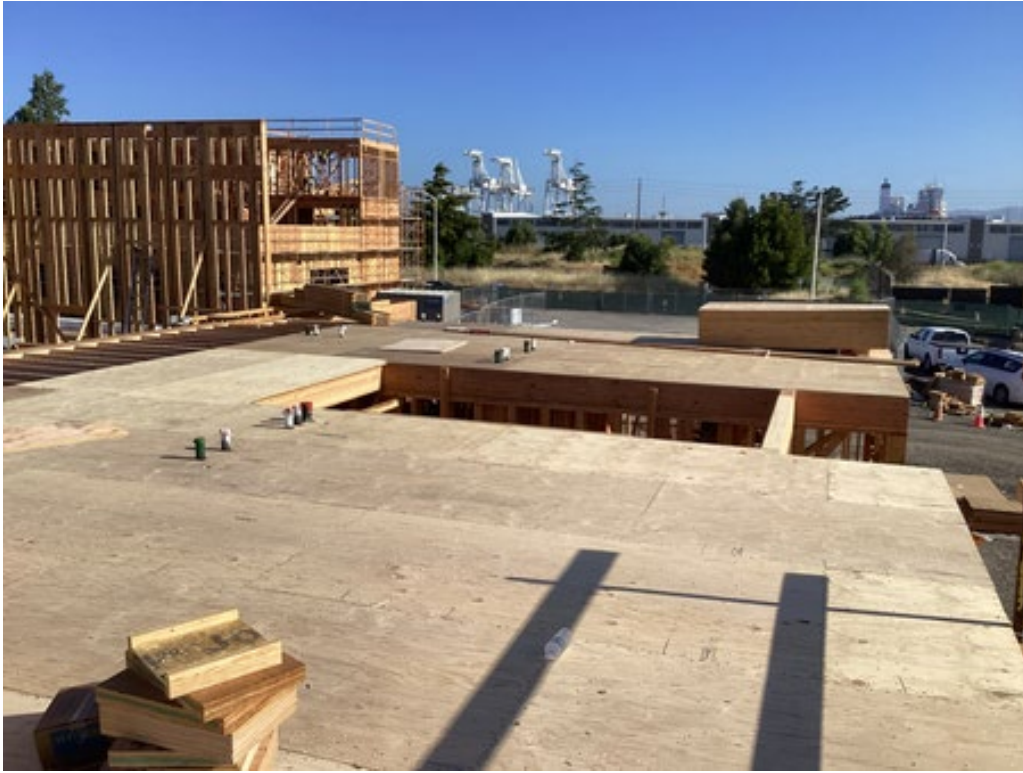
Figure 2: Subfloor Installation at Level 2
