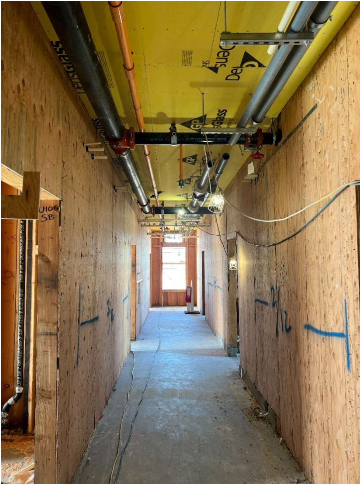
Plumbing lines, water lines, and fire sprinkler system being installed in the hallway.
