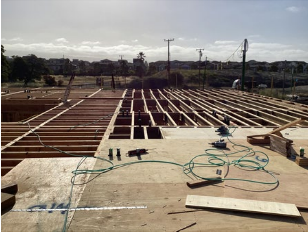
Figure 4: Joist installation at units
