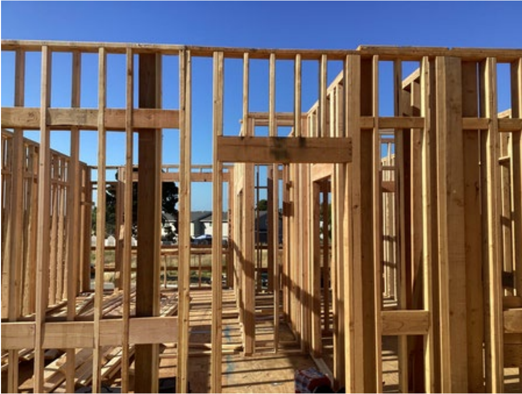
Figure 1: Walls going up at Level 2
