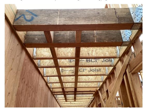
Figure 6: Photo of joists and beam installation
