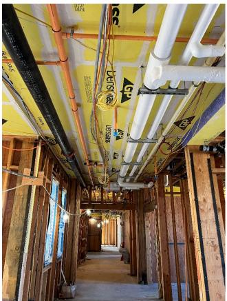
Rough plumbing, rough electrical, and fire sprinkler system installed in the hallway.
