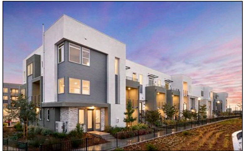
Pulte homes complex at sunset in Alameda, CA.
