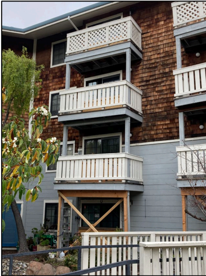
(Image left): original balconies with bracing installed prior to major work. (Image center): construction underway on resident balconies. (Image right): completed balcony replacement.
