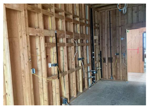
Figure 8: Rough electrical installation
