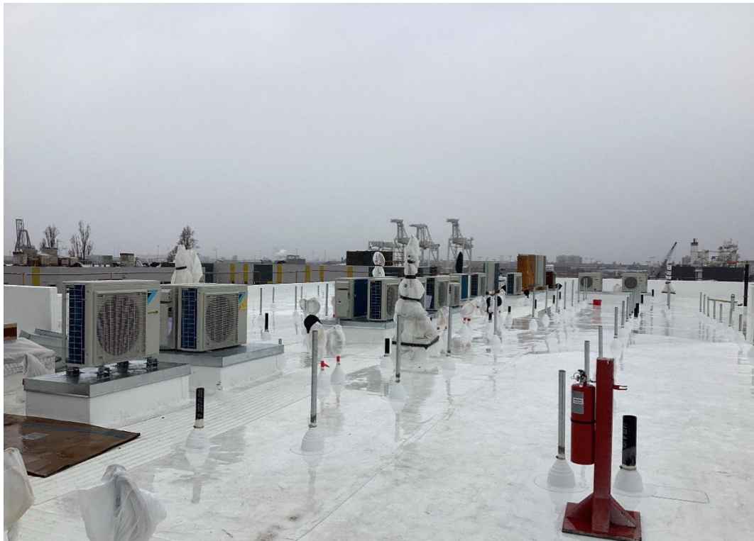
Figure 8: Installation of the heat pumps
