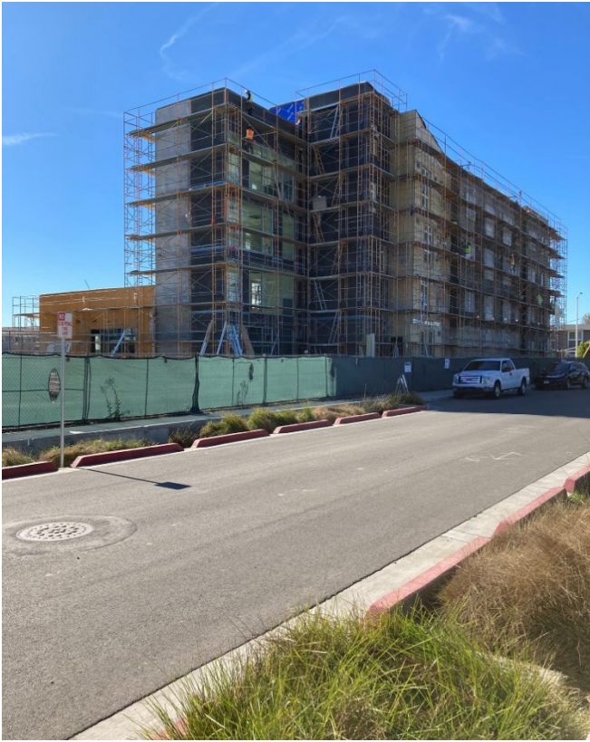
Building progress photo from northeastern elevation (view from Mosley Ave).
