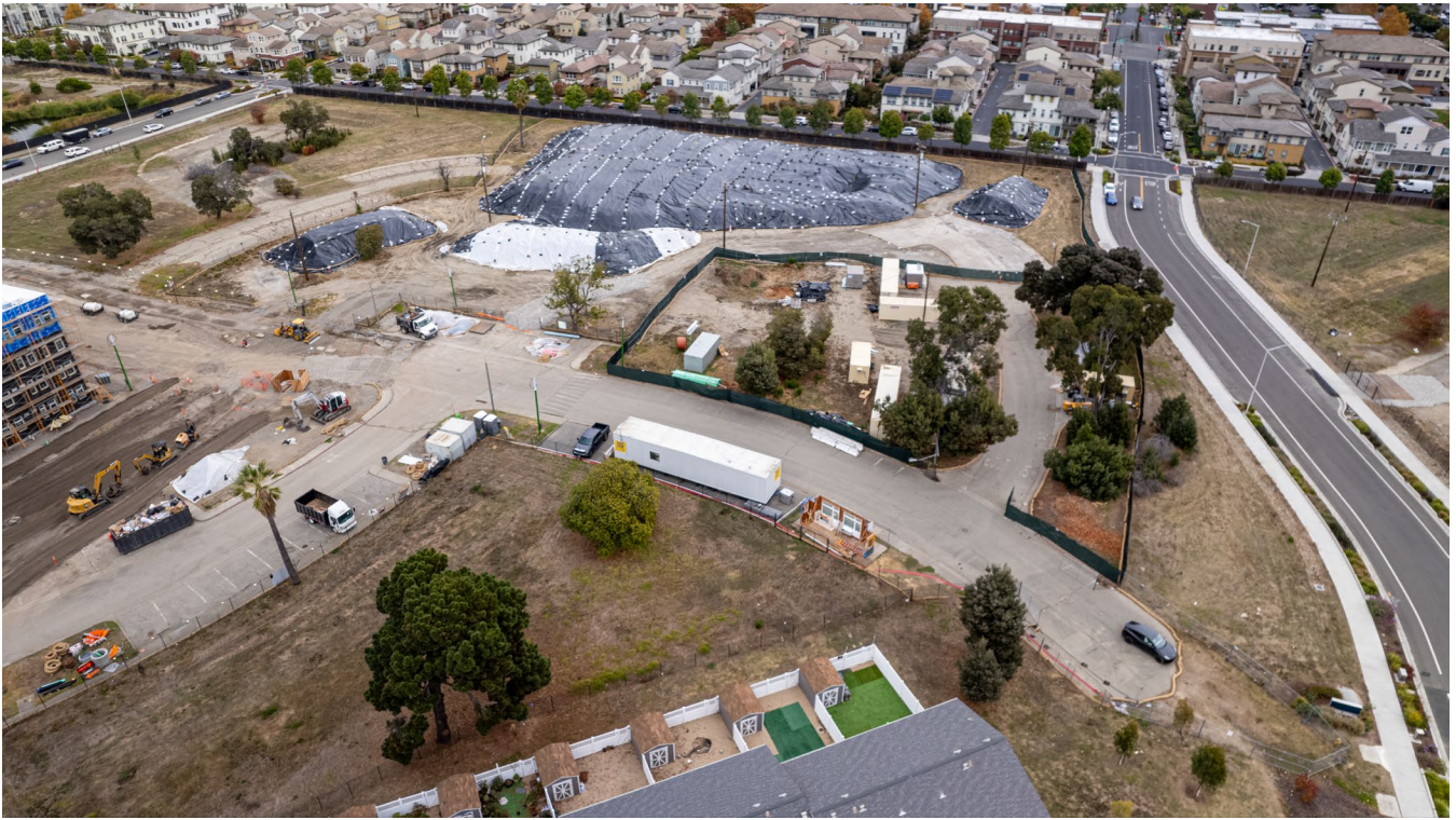
Aerial photo of the stockpile and laydown area. To the left of the photo is corner of the new Mabuhay Street and the future realignment of Lakehurst Circle at the corner of Linnet Corner.
