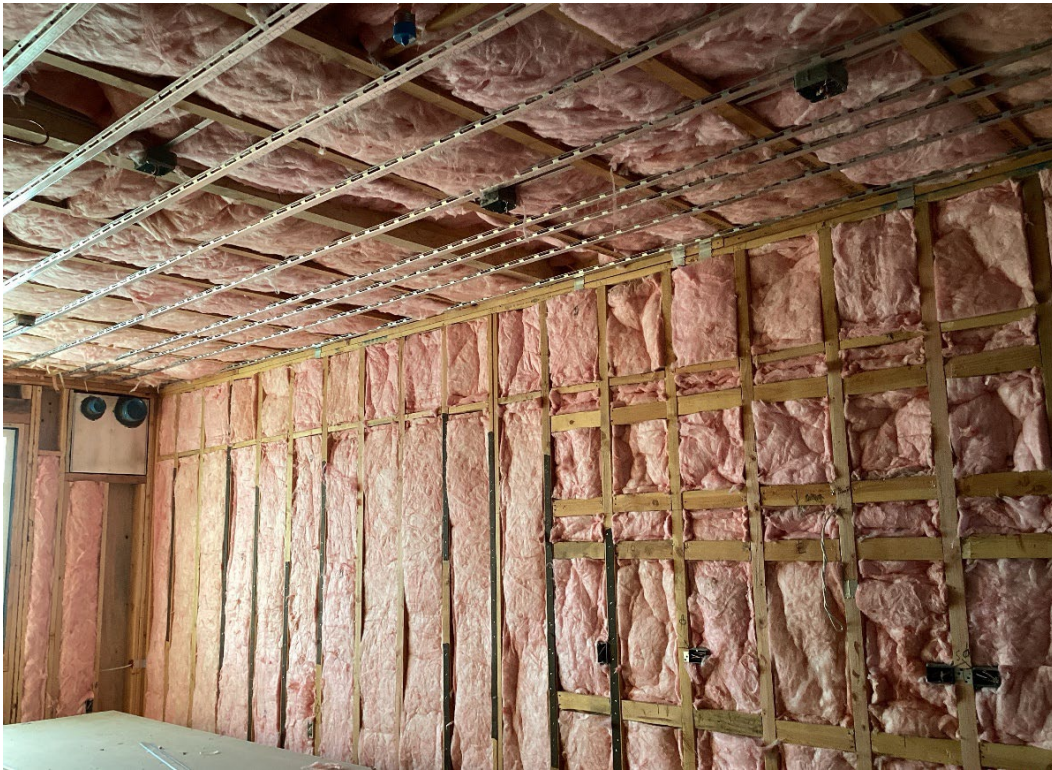
Figure 6: Installation of insulation at units
