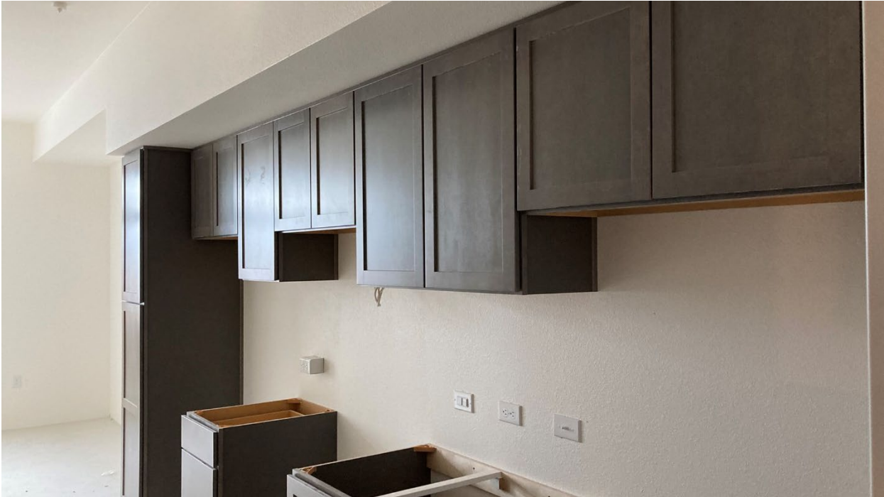
Kitchen cabinets installed at one of the units.
