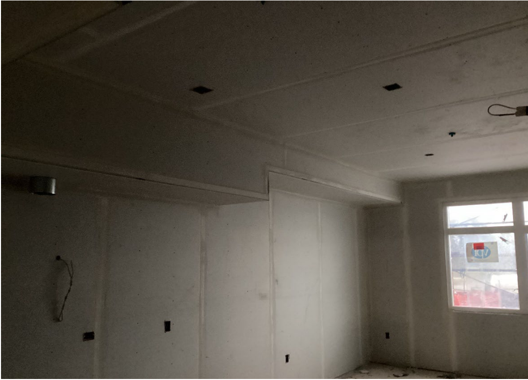
Figure 5: Completion of drywall installation at units
