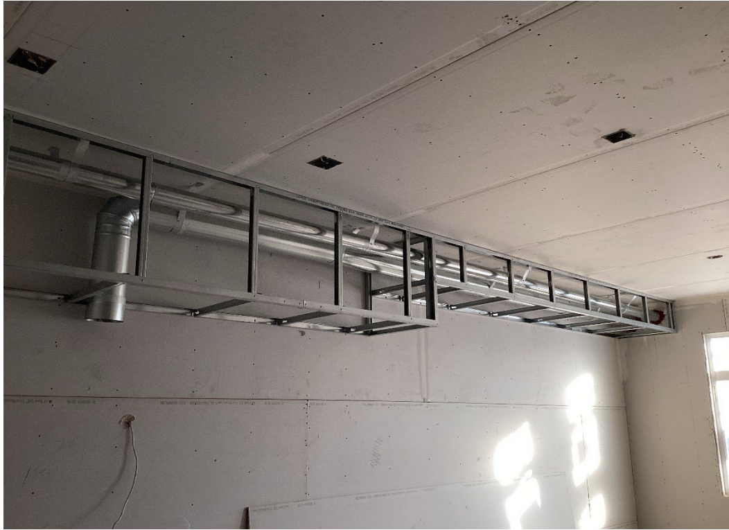
Figure 7: Completion of MEP Installation at units
